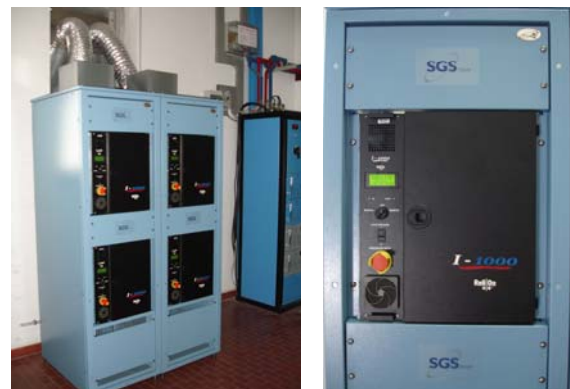
Figure 5: Mattarello's fuel cell systems.
