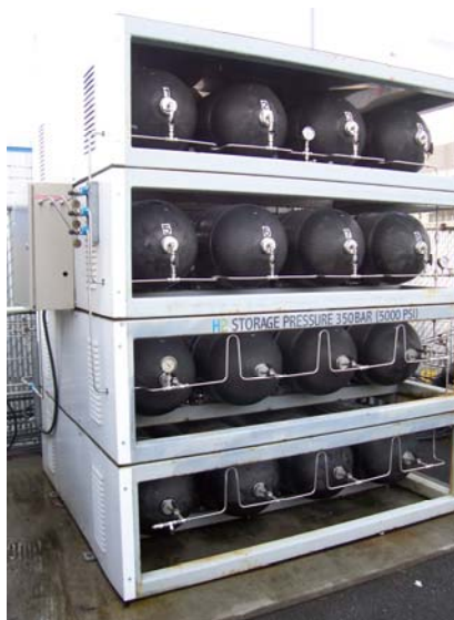
Figure 4. Dynetek 5,000 psi (350 bar) Composite Pressure Vessels In Fixed Storage Service Source: ReliOn
